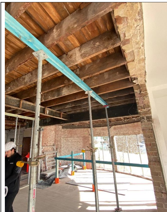
Figure 13. Original timber and steel floor structures and decking. (Source: GML, September 2024)
