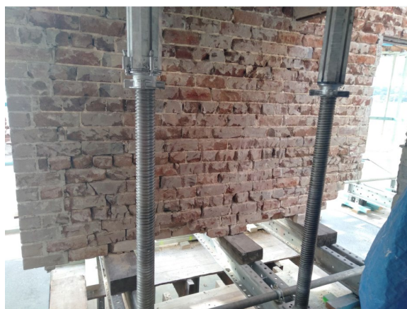
Figure 4.25 Section of wall partly removed, with temporary supports. (Source: GML, July 2024)
